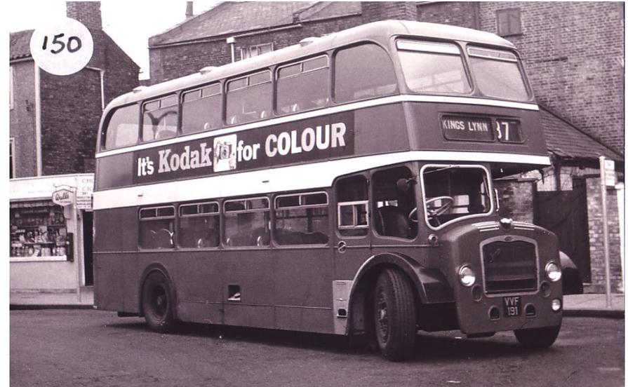
**LKD 191** (VVF 191) is seen here in the old King's Lynn Millfleet bus station, working on a local town service in the early 1960s. A total of 26 VVF registered LD5G Lodekkas seating 60 passengers were delivered to ECOC during 1957 and 1958. LKD 191 was one of the batch of nine delivered in 1957. She was withdrawn in 1975 after 18 years loyal passenger service.
