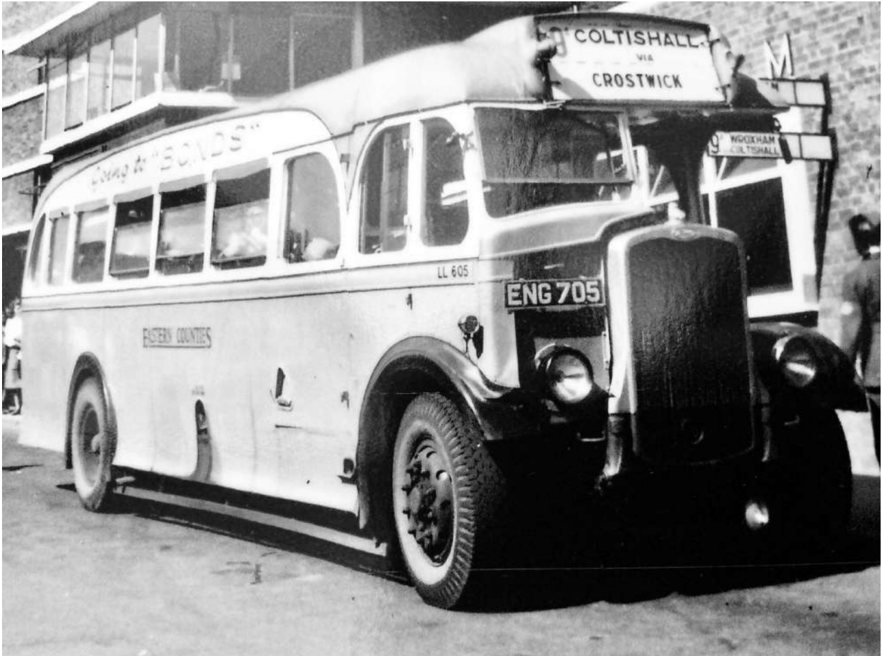
A Bristol L5G 'ordinary' single decker. 1942 - 1957. Earlier versions of the above were in the CNG registration range and were fitted with 4 cylinder engines and these models were designated L4G and were introduced in 1938 and phased out in the very early fifties.
