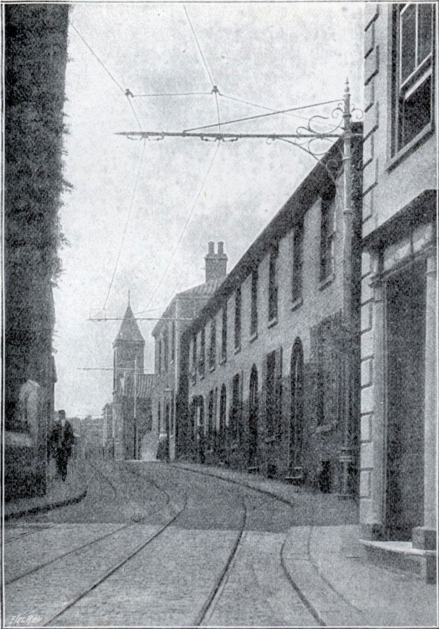
THEATRE STREET : SIDE-POLE SUSPENSION.
