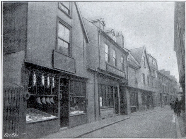
RED LION STREET BEFORE WIDENING.
